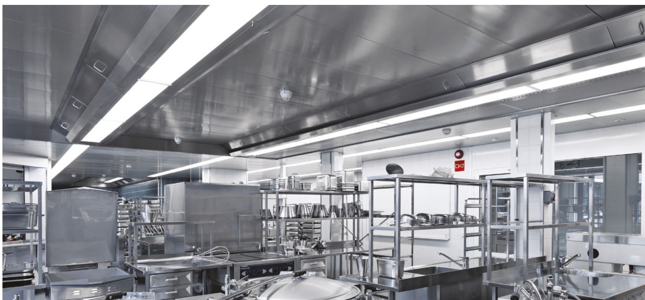
Kotka central kitchen (Kotka, Finland)
