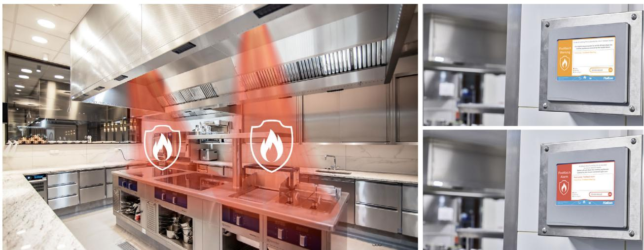
**Stage 1 alarm** - A warning is displayed on Halton Touch Screen. It is relayed with light signal and buzzer fitted on the front of the hoods.
